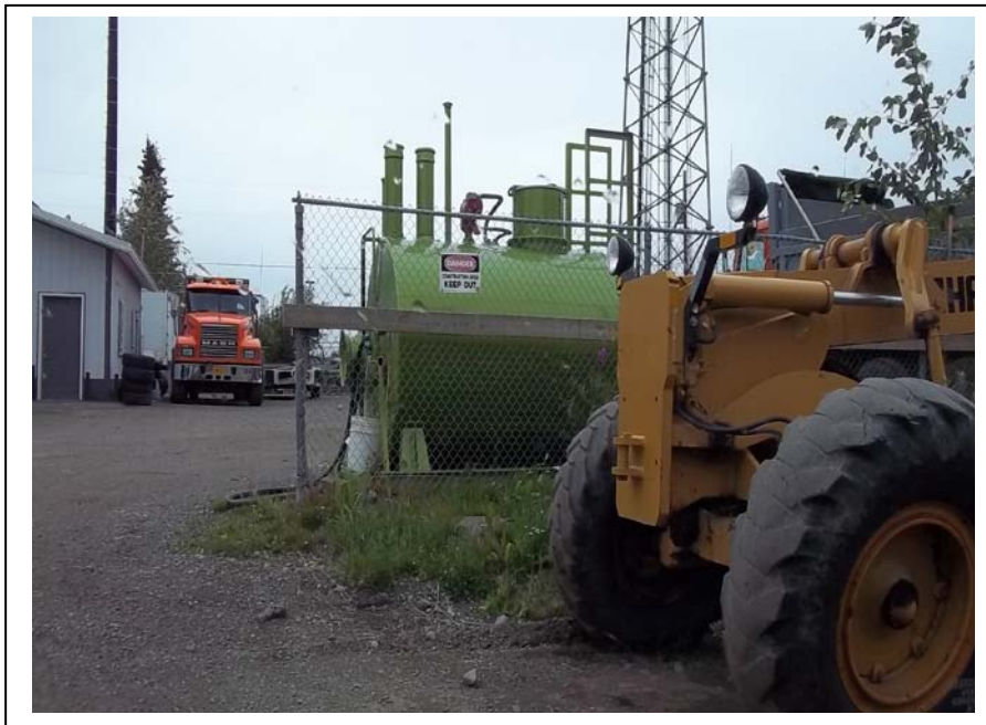
Photo 18: The above ground storage tank located on Talkeetna Street. (August 3, 2011)
