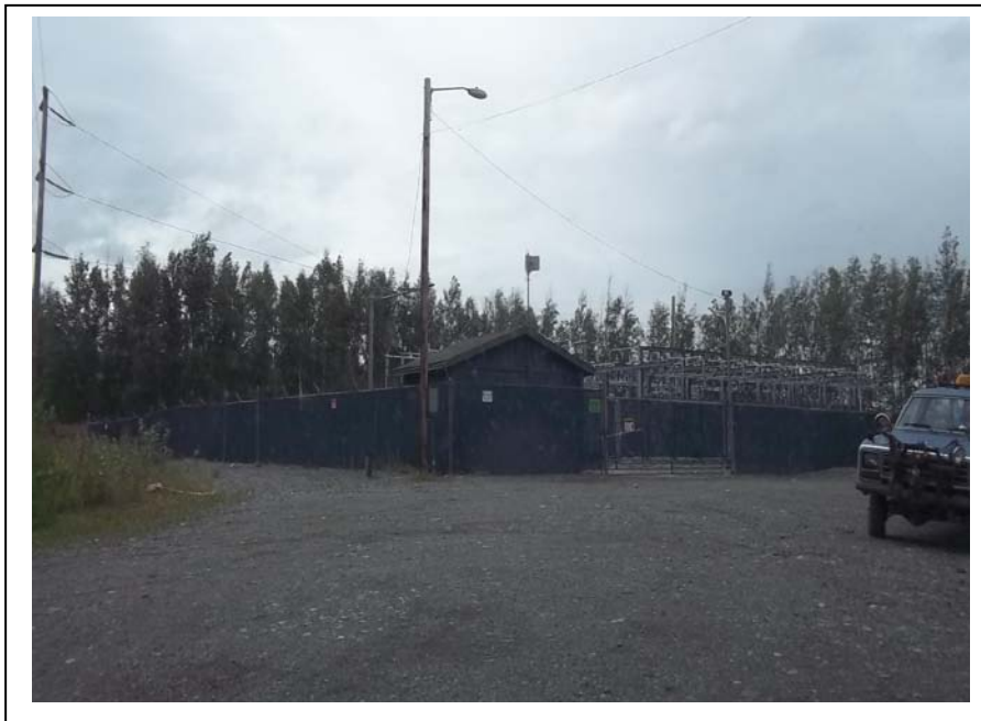
Photo 14: The MEA substation located at the end of Denali Street, adjacent east of the Talkeetna/Yenlo Corridor. (August 3, 2011)
