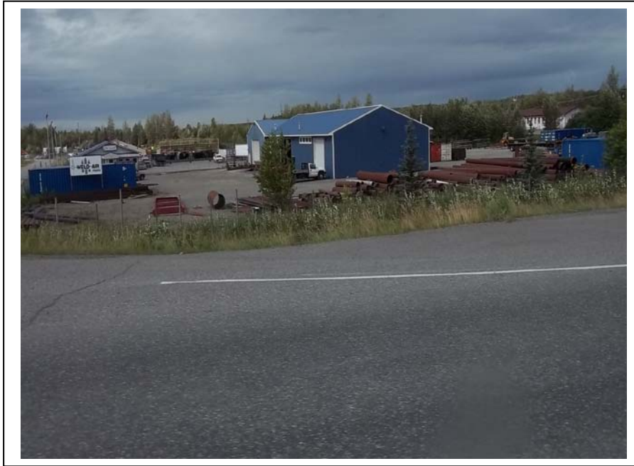
Photo 7: The Weld Air facility located adjacent west of KGB Road. (August 3, 2011)
